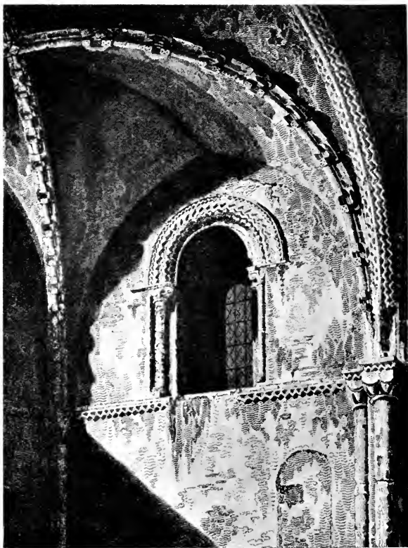
FIG. 31. VAULT OF CHANCEL, S. PETER'S Showing Norman ribs with enrichments.
